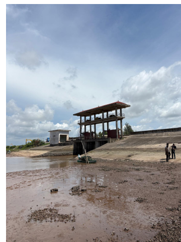
Figure 3.5: Gate 10 in Dike Ring 3 (Authors, 2025)
