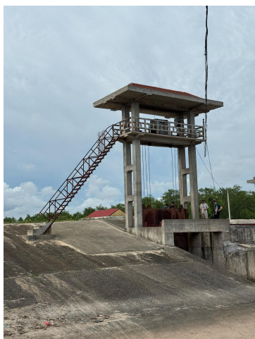
Figure 3.3: Gate in Dike 4 (Authors, 2025)
