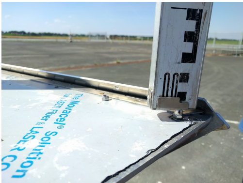
Figure 6.15: Close up of the bolt rod connection
