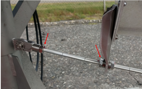
Figure 6.22: The rigger construction for reflector alignment. The distance between the bolts that have been highlighted should be measured.
