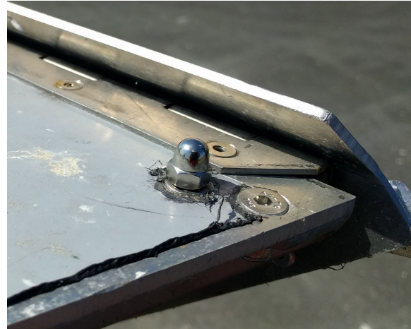
Figure 6.21: Levelling marker after changing bolts.
