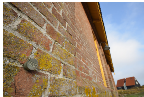
Figure 2.7: Example of a NAP control point, Vlissingen, NL. (Photo D.Bruin)
