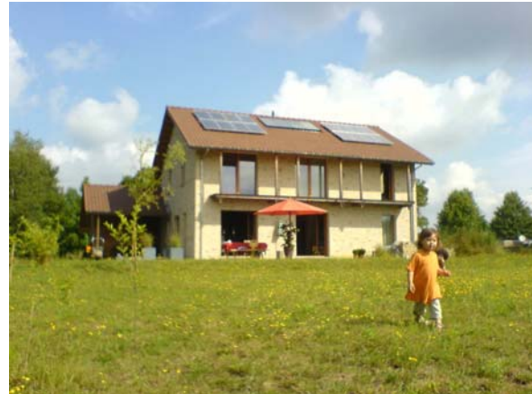
Figure 1: Passive house in Heusden-Zolder (mind the shade on the walls: in mid summer the windows do not receive direct sunlight)
