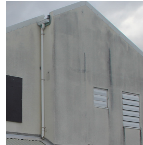
Useless roof gutter
