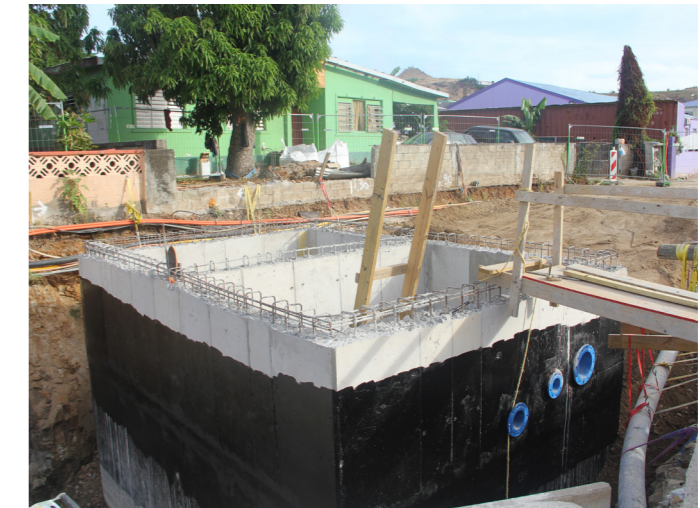
Wastewater tanks under construction
