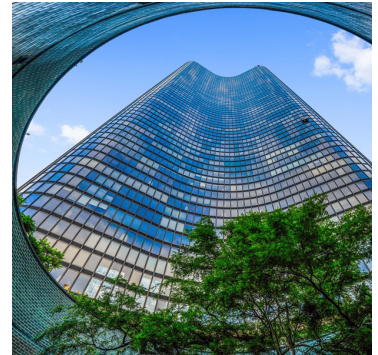
106 View of tower from inner rotunda (Chicago Top Condos, 2018)
