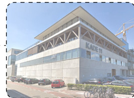
KADE 11 Current function | Office State of building | Excellent
