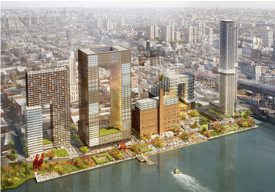
34 Domino Sugar Factory redevelopment (Schulz, 2016)
