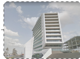
DANZIGERKADE 181 Current function | Office State of building | Excellent
