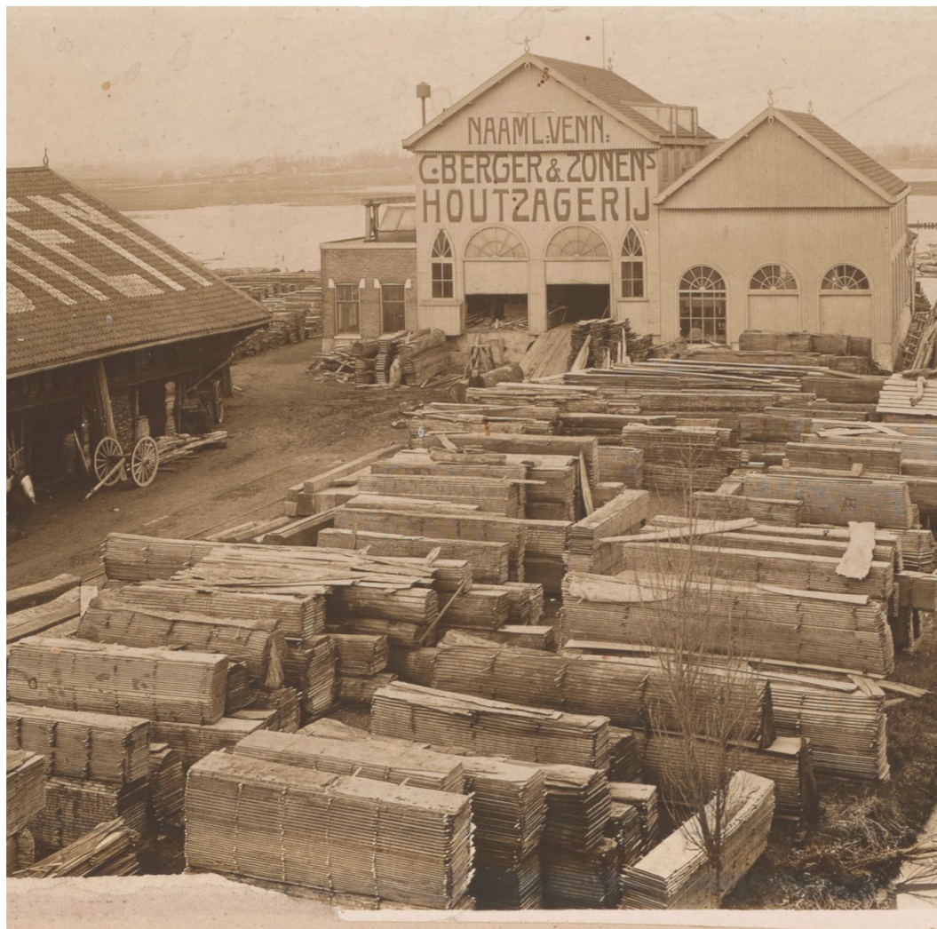
timber stacks Rotterdam Reg. Arch. Dordrecht
