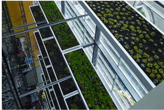
Figure 3 Planters in second skin façade (Copijn, n.d.)
