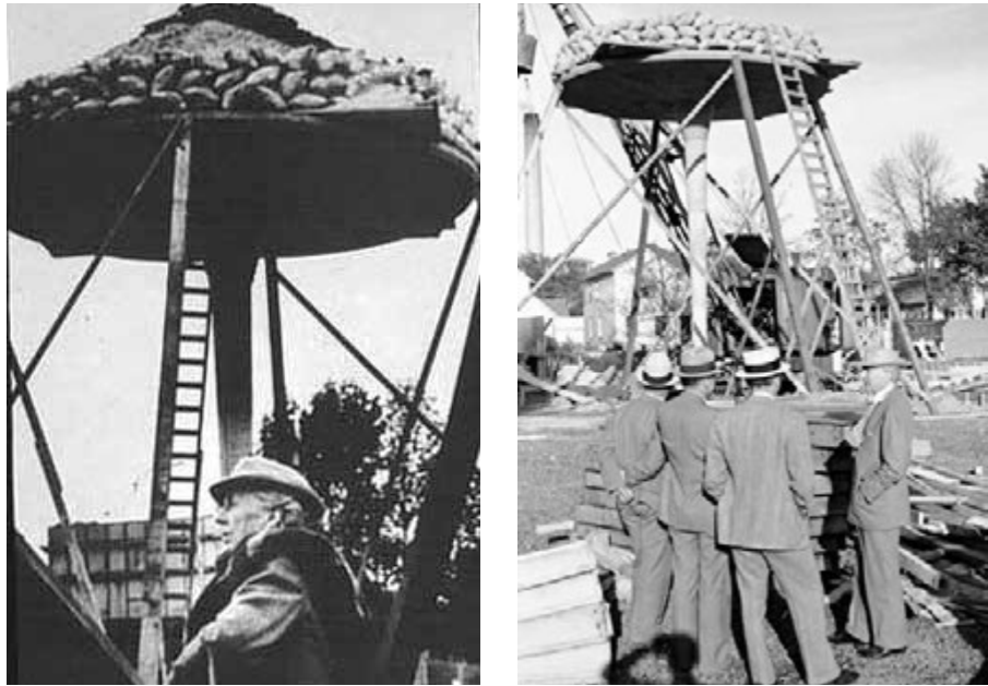
FIG. 5.7 Frank Lloyd Wright nonchalantly conversing in front of the heavily overloaded columns of the SC Johnson Administration Building. [Courtesy SC Johnson].
