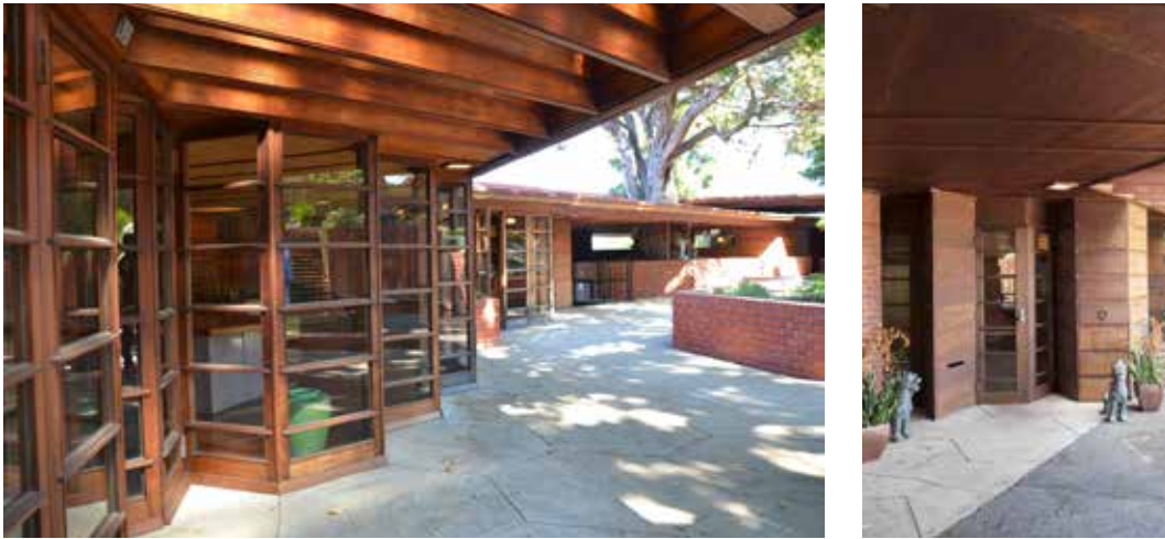
FIG. 5.6 Hanna House. Left: window sash in the kitchen area. Right: 'virtuoso folds' in the entrance area. [Photos: Regis Vincent]
