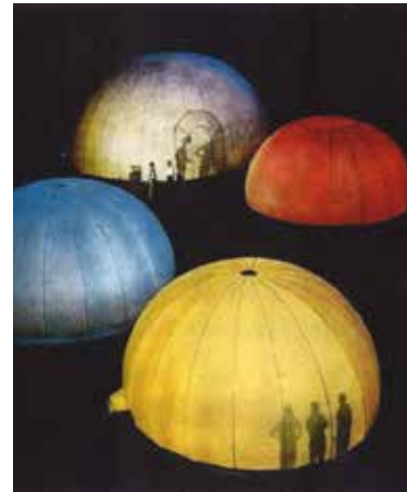
FIG. 4.37 Fiberthin Airhouses at a Kentucky university. Photo originally appeared in November 11, 1957 issue of Life magazine.
