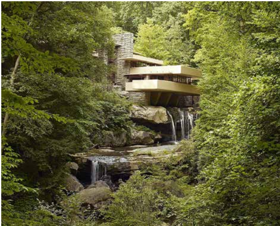
FIG. 3.24 Rock ledges around the house Fallingwater. [Photo: Carol M. Highsmith, Library of Congress]
