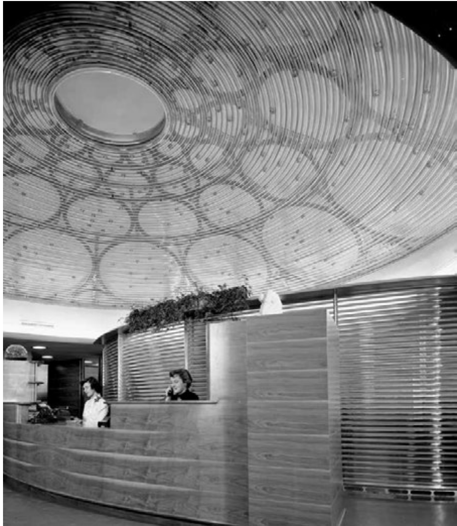
FIG. 1.24 SC Johnson Administration Building, advertisement department, cupola and screen of Pyrex tubes. [Courtesy of SC Johnson]
