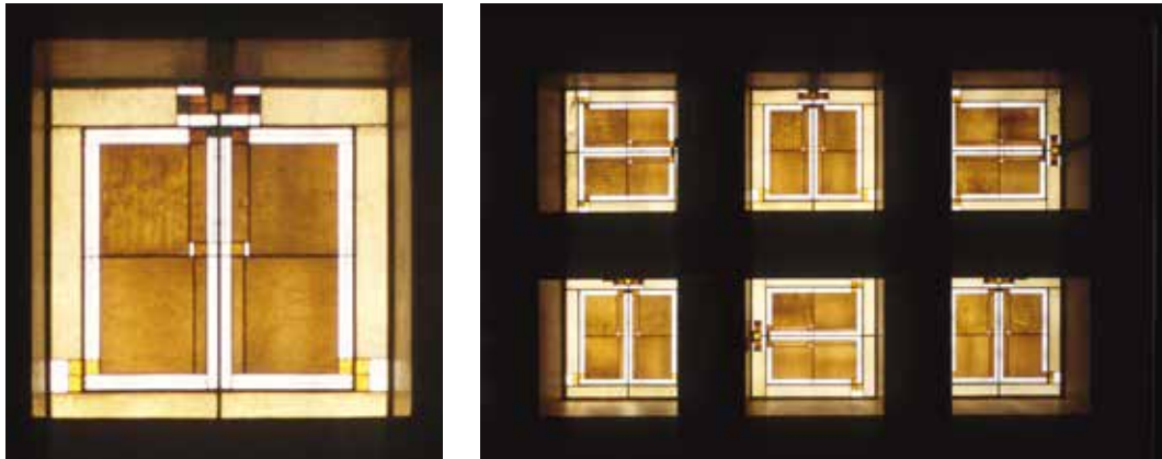
FIG. 1.4 Unity Temple, skylights. Pattern of the leaded glass in one coffer and in a series of coffers. [Photo: Frans Sturkenboom]
