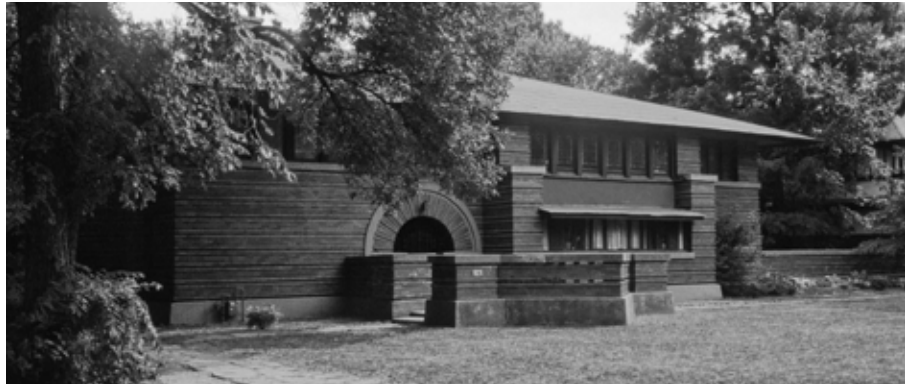
FIG. 2.19 Heurtley House, Chicago (IL), 1902. Ornamental bastion before the front door. [Photo: Frans Sturkenboom]
