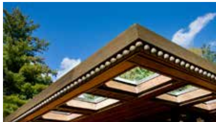
FIG. 2.38 Weltzheimer House, Oberlin, Ohio, 1948. Perforated eave with cornice. [Photo: Patrick Kilkenny]
