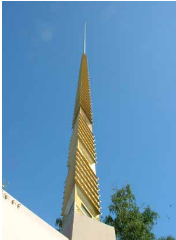
FIG. 1.36 Antenna on the Marin County Civic Center. [Photo: User: nandhp, CC-BY-SA 2.5 generic]
