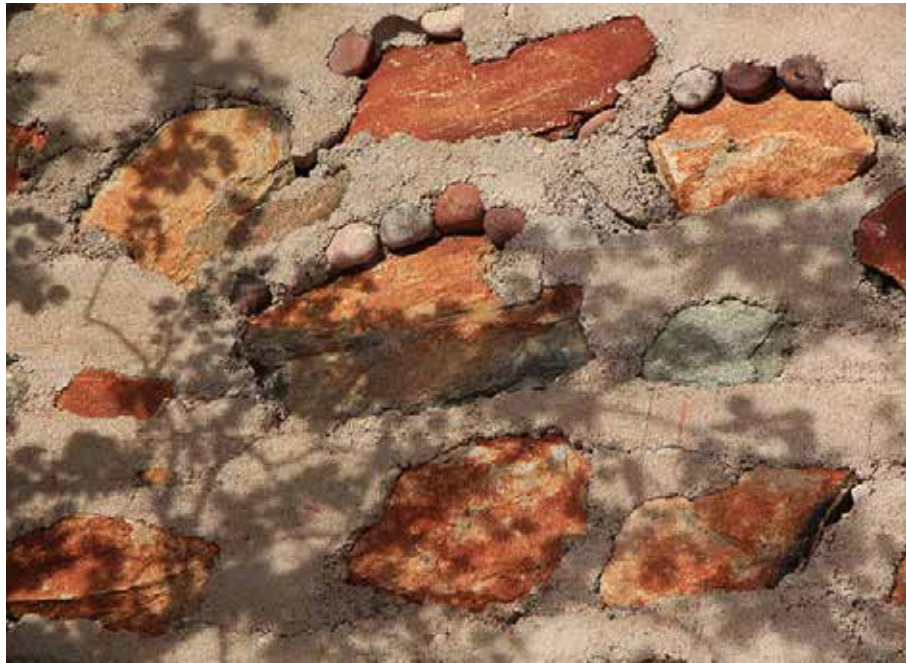
FIG. 4.18 Taliesin West, Scottsdale (AZ), 1937: desert concrete. [Photo: Steven C. Price; CC BY-SA 4.0]
