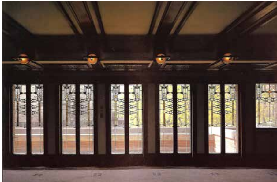
FIG. 2.20 Robie House, terrace doors with coloured leaded glass. [Photo: © Yukio Futagawa]
