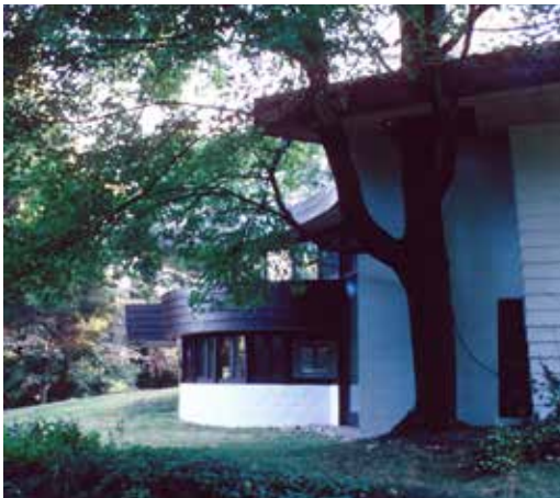
FIG. 1.49 The concave side of the Curtis Meyer House. [Photo: Frans Sturkenboom]
