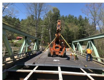
(b) Replacement of Rugg Bridge deck (US), originally built in 1938 [Composite Advantage, 2018].
