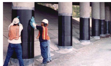
(c) Wrapping of concrete column [Hamakareem, -].
