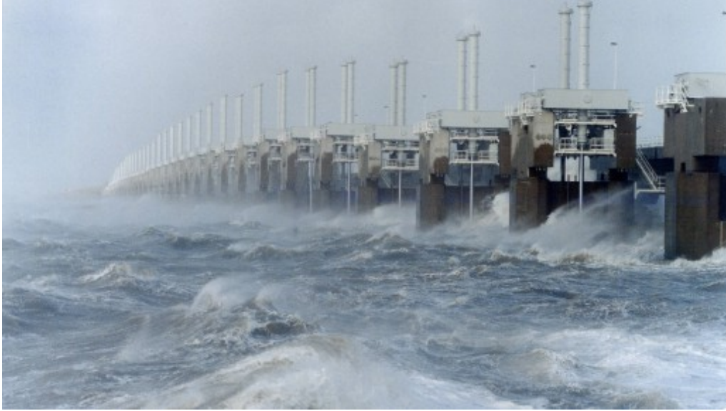
Figure 1.2: Eastern Scheldt storm surge barrier (Watnoodsmuseum, 2018)
