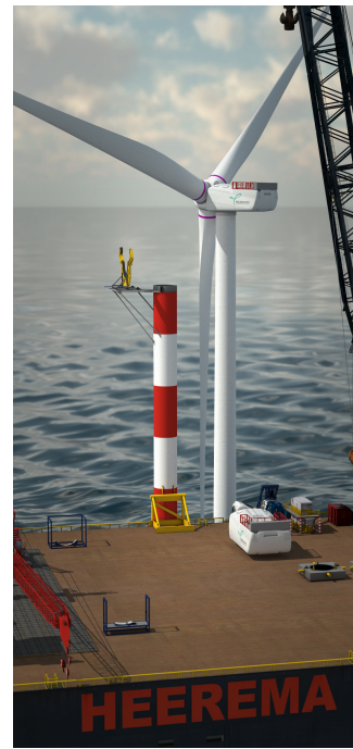
Figure 1.6: RNA installed on turbine tower (Heerema Marine Contractors, 2020a)
