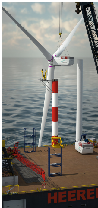
Figure 1.5: RNA lift from vessel to turbine tower (Heerema Marine Contractors, 2020a)
