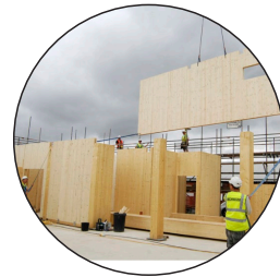
CLT Timber construction
