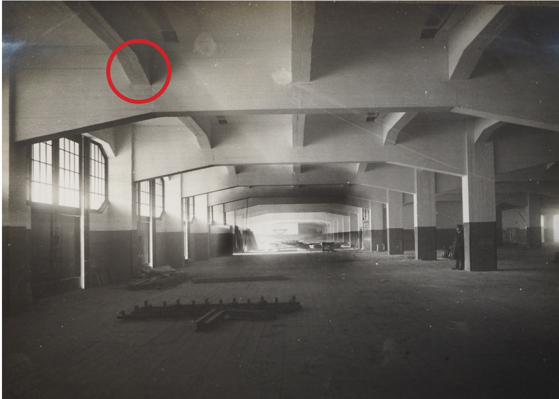
Original roof structure girder and beam are connected influenced by Hennebique system
