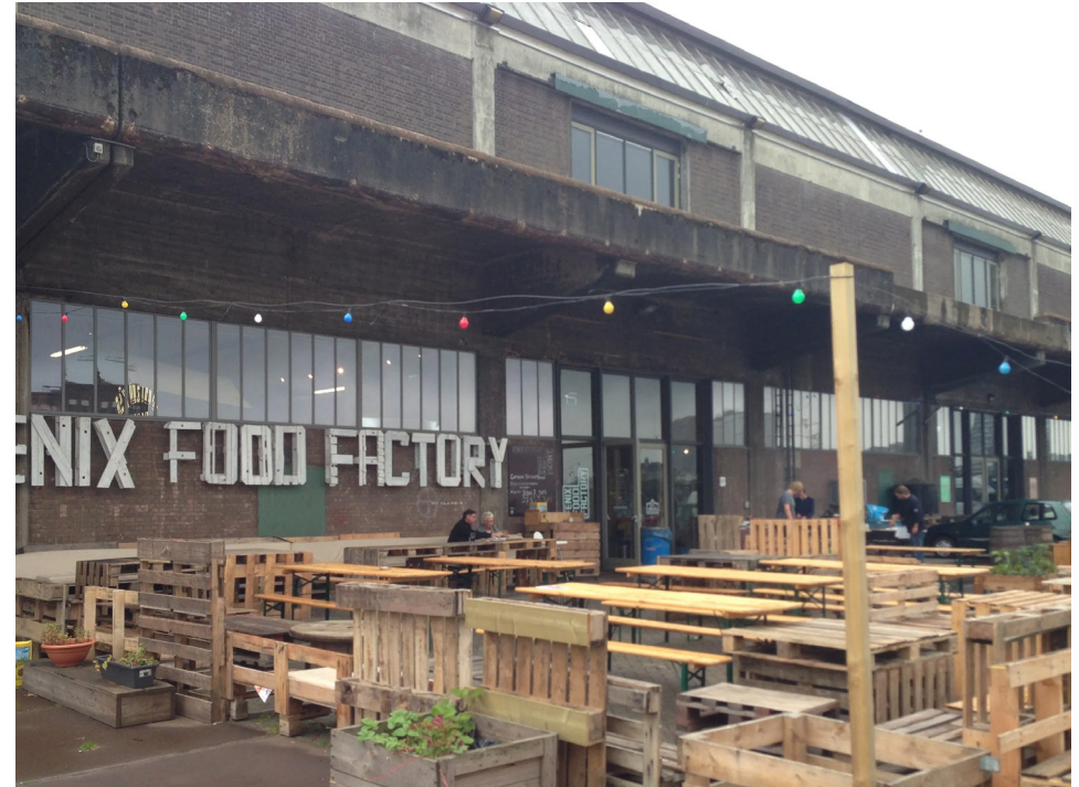
current north facade
