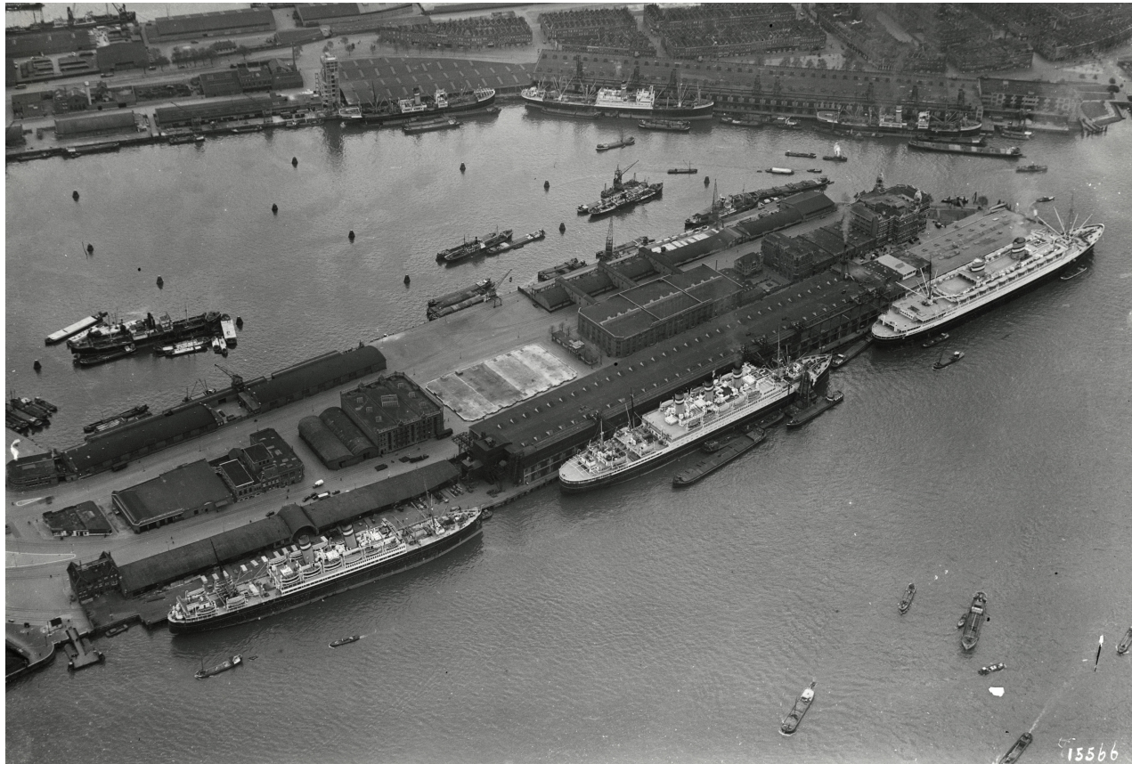
Loods San Francisco The biggest storage in the world at the time
