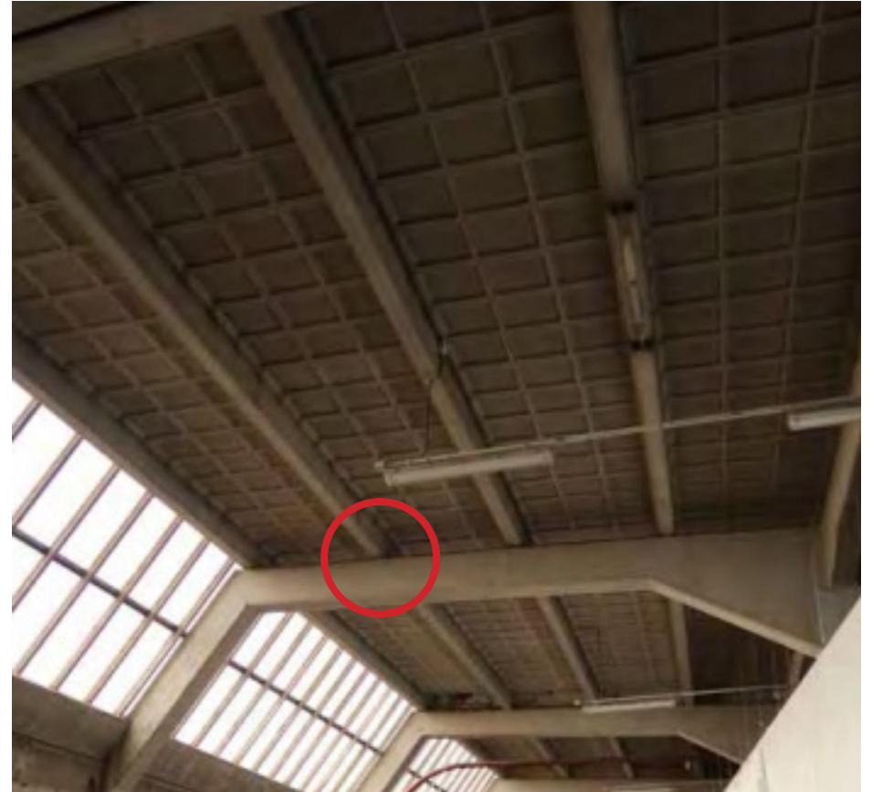
New roof structure beam on girder
