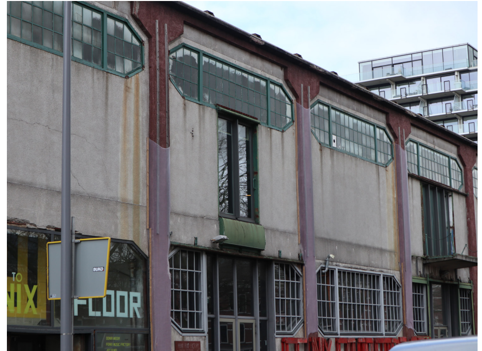
current south facade
