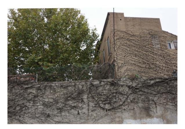
Fig. 31: Roots spreading accross the wall, increasing it's porosity
