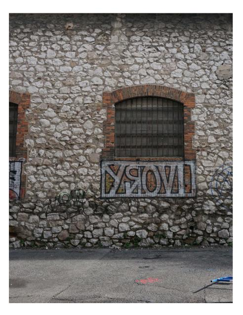
Fig. 28: Algal growth on limestone wall - uneven vertical distribution.
