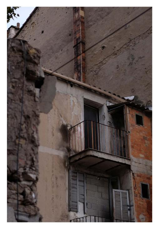
Fig. 20: Material assemblage - brick, concrete, metal and limestone.
