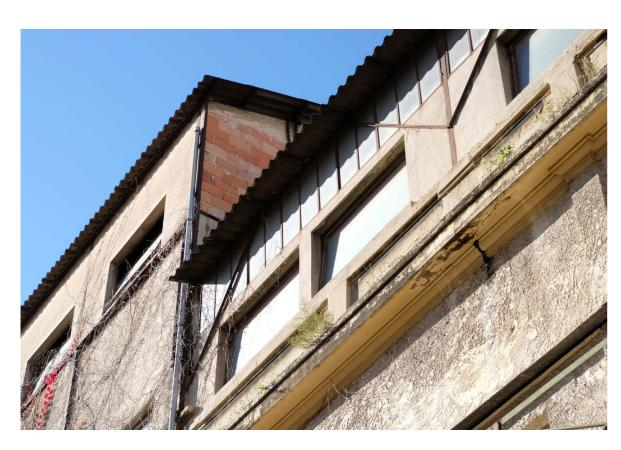
Fig. 21:Material assemblage - brick, concrete, metal and glass.
