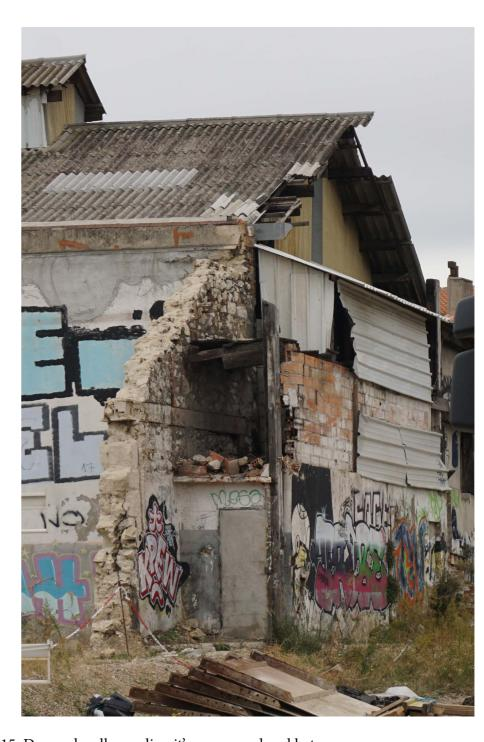
Fig. 15: Decayed wall revealing it's compound and heterogenous character
