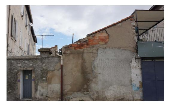
Fig. 22: Layering of materials as a result of decay.
