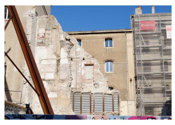
Fig. 18: Fragility revealed by half collapsed wall, supported by various metal prosthesis.
