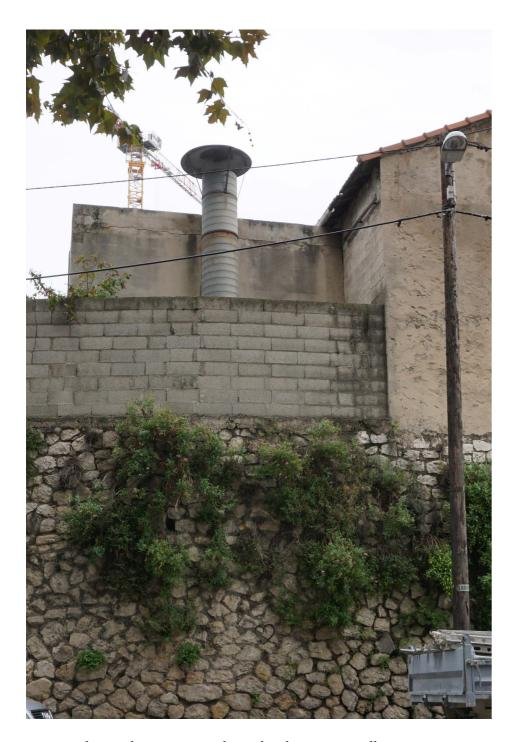
Fig. 30: Plants adopting to cracks within limestone wall.
