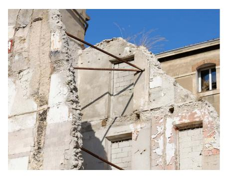
Fig. 7: Metal protesis applied to decayed wall
