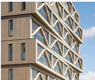
Patch 22, a hybrid timber building features a glulam post beam structure with a demountable prefab concrete flooring system. Design: FRANTZEN et al. Picture: Luuk Kramer
