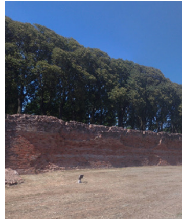
Figure 16: The walls of Ferrara from the outside, which are higher and end abruptly (Google Streetview, 2019)
