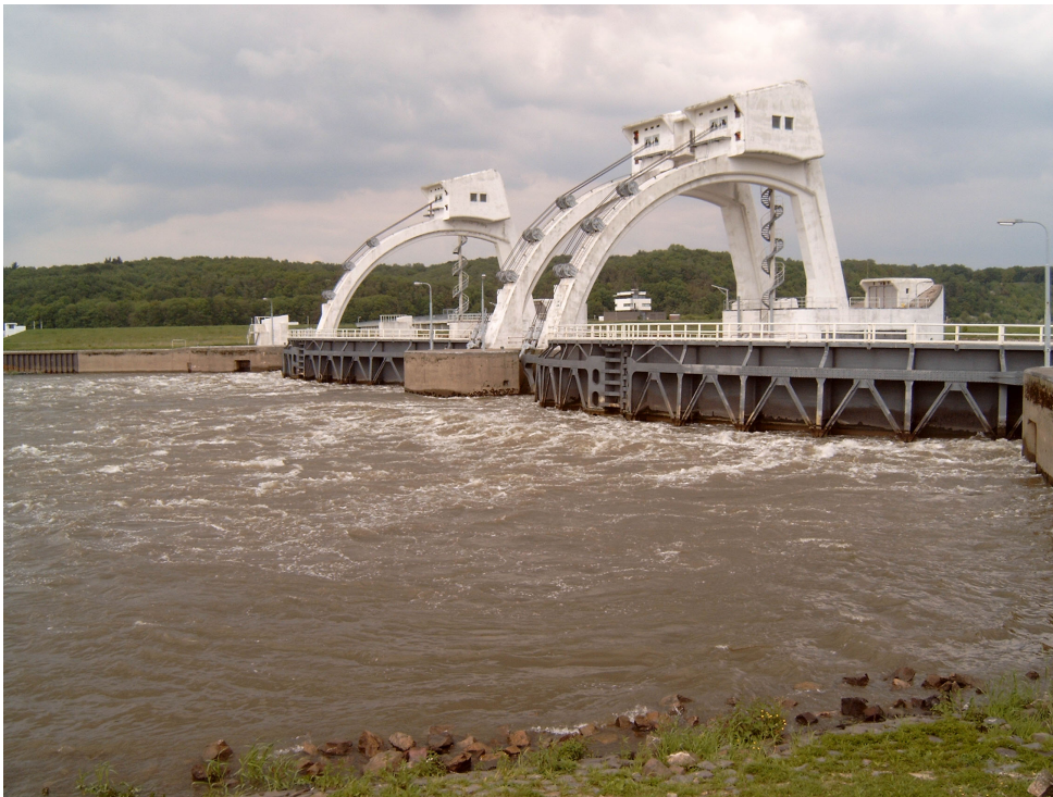
FIGURE 1.1 The weirs of the sluice and weir complex near Driel in the river Nederrijn (The Netherlands) are examples of a hydraulic structure with a considerably increased turbulence level downstream of it and hence an increased flow attack on the bottom in this region.
