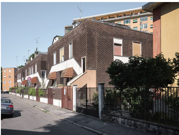
Fig. 2.31 QT8 residential buildings (Domus, 2022)
