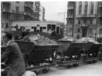
Fig. 1.3 Decauville used for the removal of rubble (Unknown, 1945)
