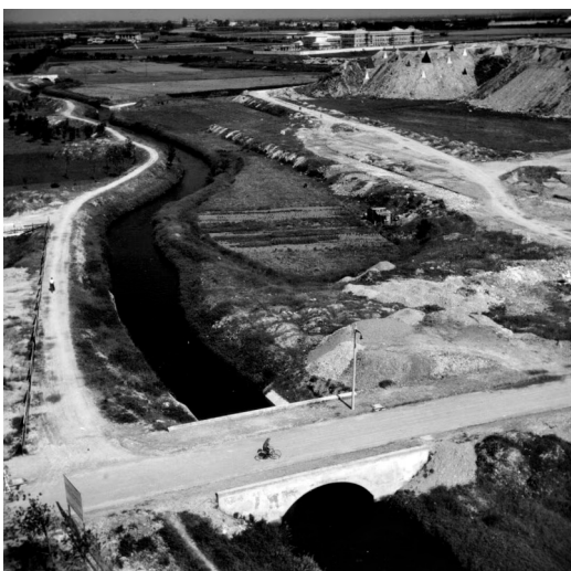
Fig. 2.11 Working site for the Monte Stella (Archivio Piero Bottoni, 1948)
