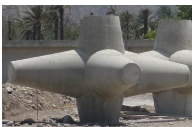
Figure 1-1: First Crablock shape with 2 short hubs [Hendrikse, 2014]
