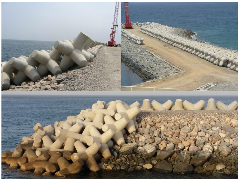
Figure 1-3: Use of Crablock on the breakwater in Al Fujeirah [Hendrikse, 2014]
