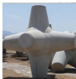
Figure 1-2: Current 3D symmetrical shape of Crablock with fillets [Hendrikse, 2014]
