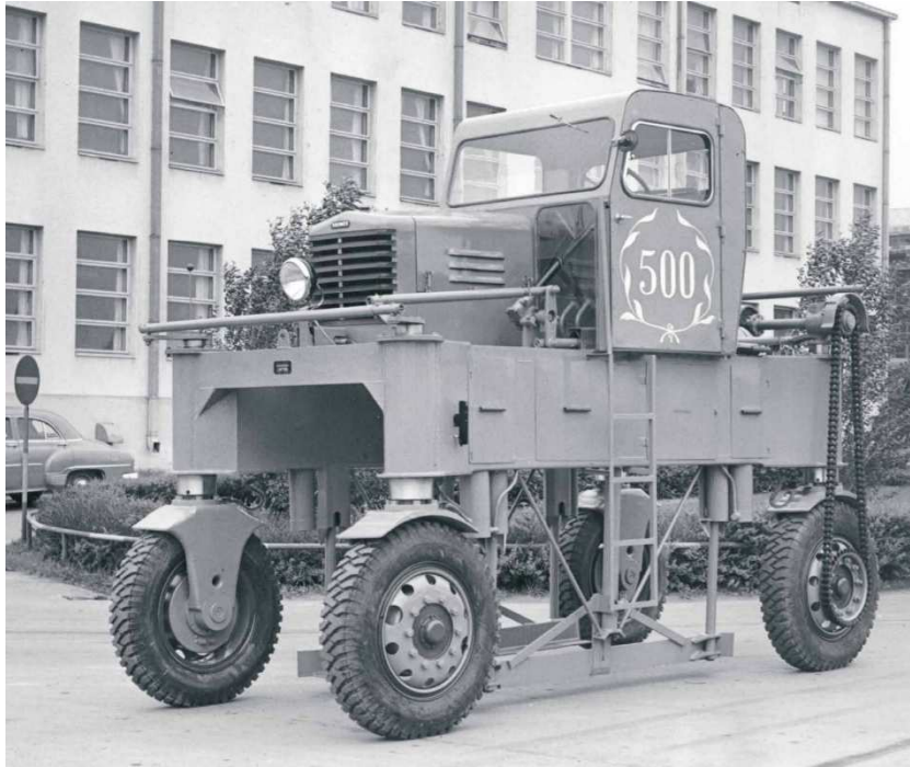
Figure 9 - Ancestor of the modern container straddle carrier (source: Kalmar )
