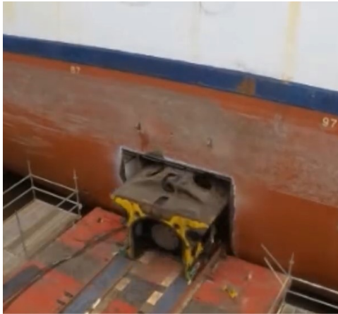
(a) Engine removal via rails (MAN ES, 2020)
