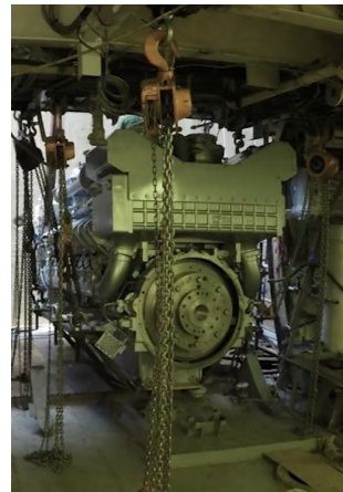
(b) Engine installation with C&T (Amico & Co, 2024)
