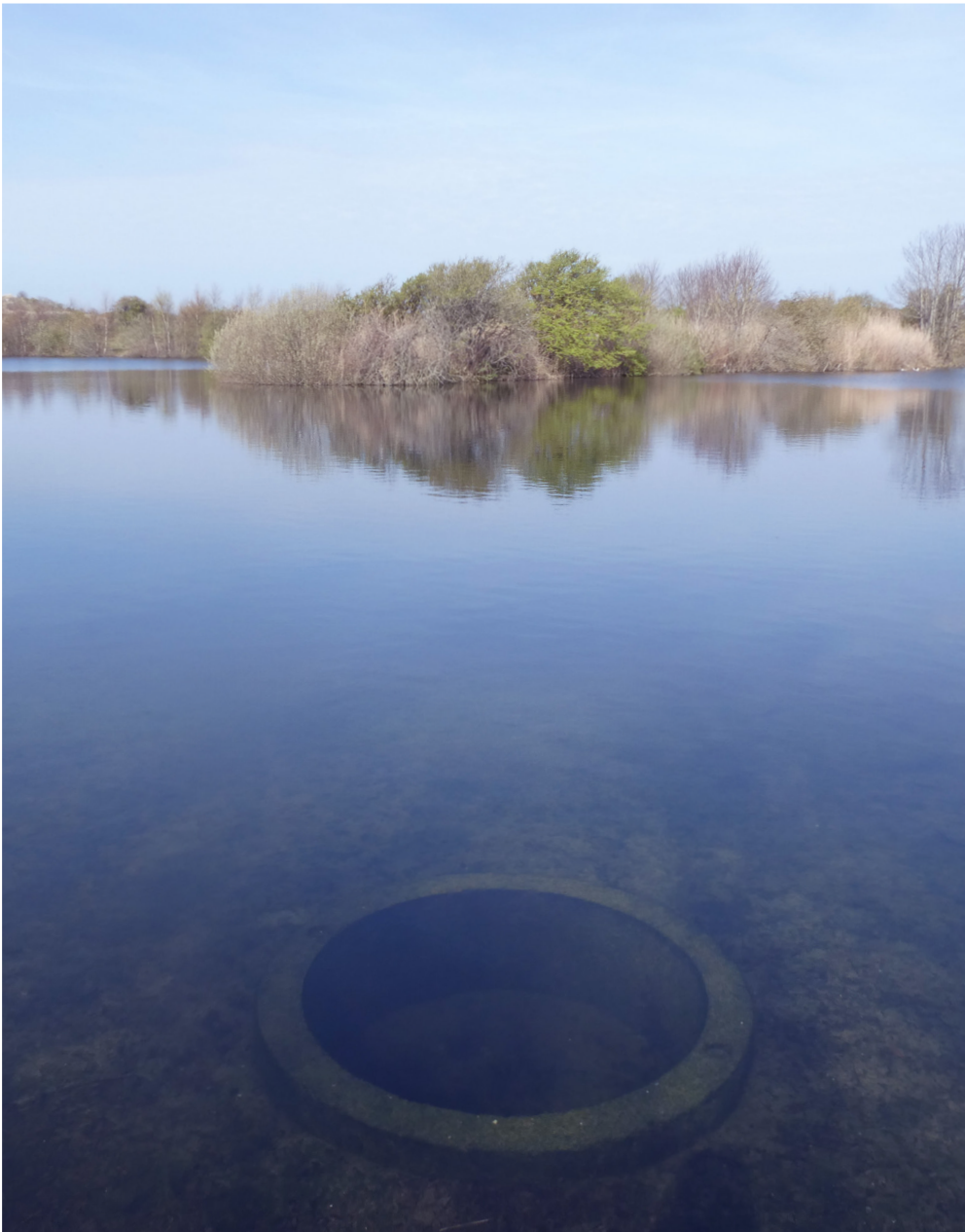
Figure 2: An infiltration lake, including a pipeline transporting freshwater to the dune lakes.
