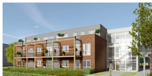
figure 16: Three-storey timber-frame residential building in Zuidwolde, The Netherlands, 2011.
