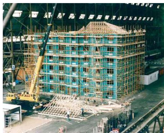
figure 20: "TF2000" research building at BRE Airship Hangar in Cardington, United Kingdom, 1999.
