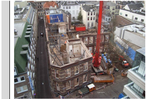
figure 24: Construction of a building in the city-centre.
