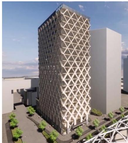
*Figure 15: Example of the diagrid structure (Moon, 2007)*
