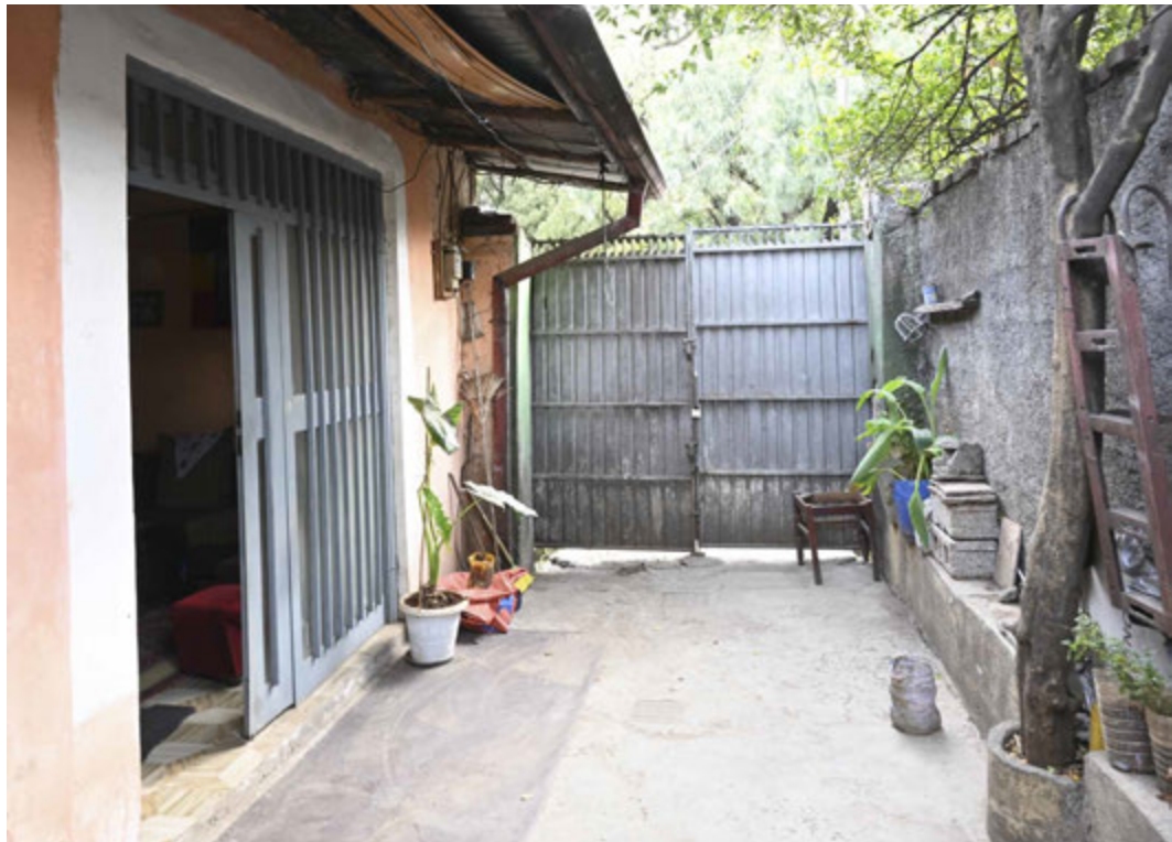
FIG. 5.6 Bizunesh's gibi and secondary access towards the side street.
