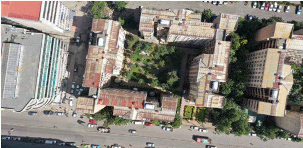
FIG. 5.30 Drone image of Lideta Condominium.
