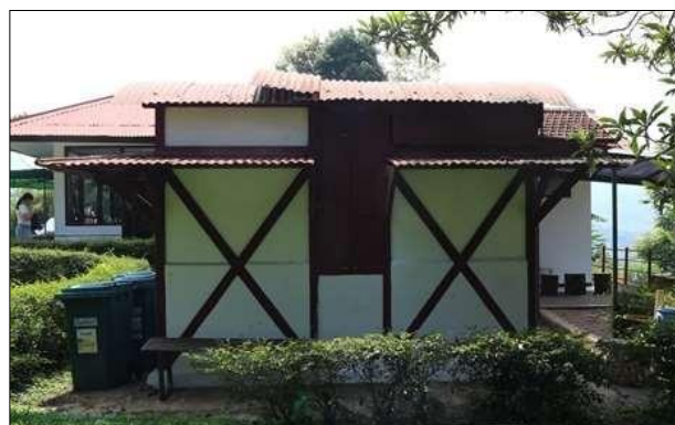
Figure 6: Condition of the transit telescope building that has been preserved, even though the telescope is no longer there and is displayed in the Exhibition Room of Bosscha Observatory. The building is seen to the East (top), and to the North (bottom), with the sliding roof visible. There is an additional roof underneath that protects the walls from direct rain (photographs: the authors).
