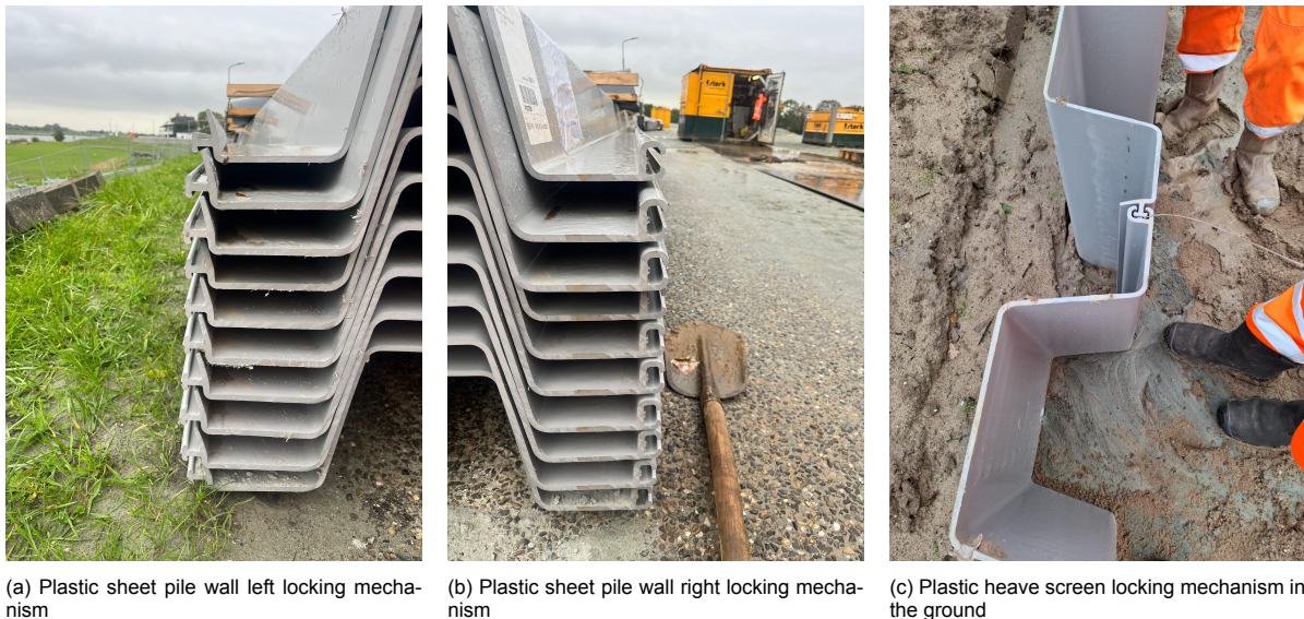
Figure 3.3: Plastic heave screen locking mechanism
