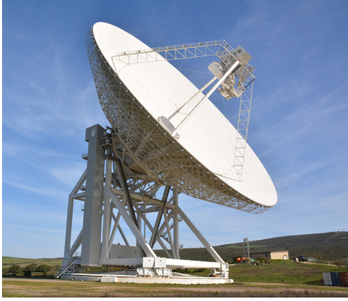
Fig. 6: Sardinia Deep Space Antenna [11]
