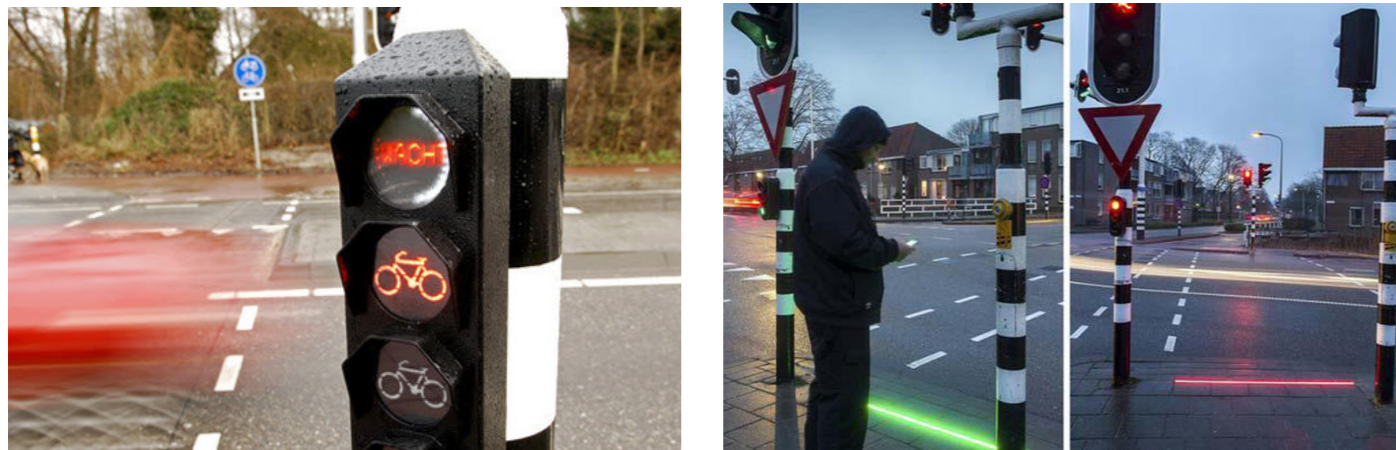
Image 13 & 14. From right to left: 1. Countdown traffic light to provide feedback while waiting, 2. Additional traffic lights in the pavement create awareness for people who are already looking down at their phones.
