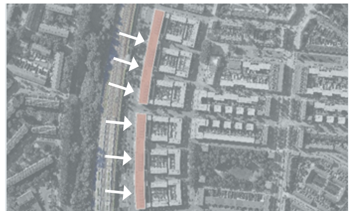
Fig 24. 272 Spoorwijk noise barrier (Own image)
