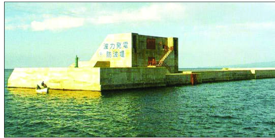
Figure A.3: Breakwater of the port of Sakata, Japan, with an integrated OWC device.
