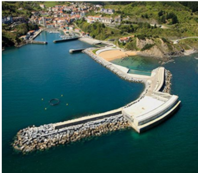
Figure 2.1: The Mutriku OWC device, integrated into the breakwater protecting the harbour. [28]
