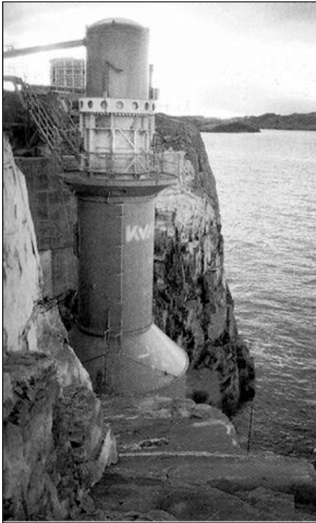
Figure A.2: The shoreline OWC device in Toftehallen, Norway, built into a cliff.
