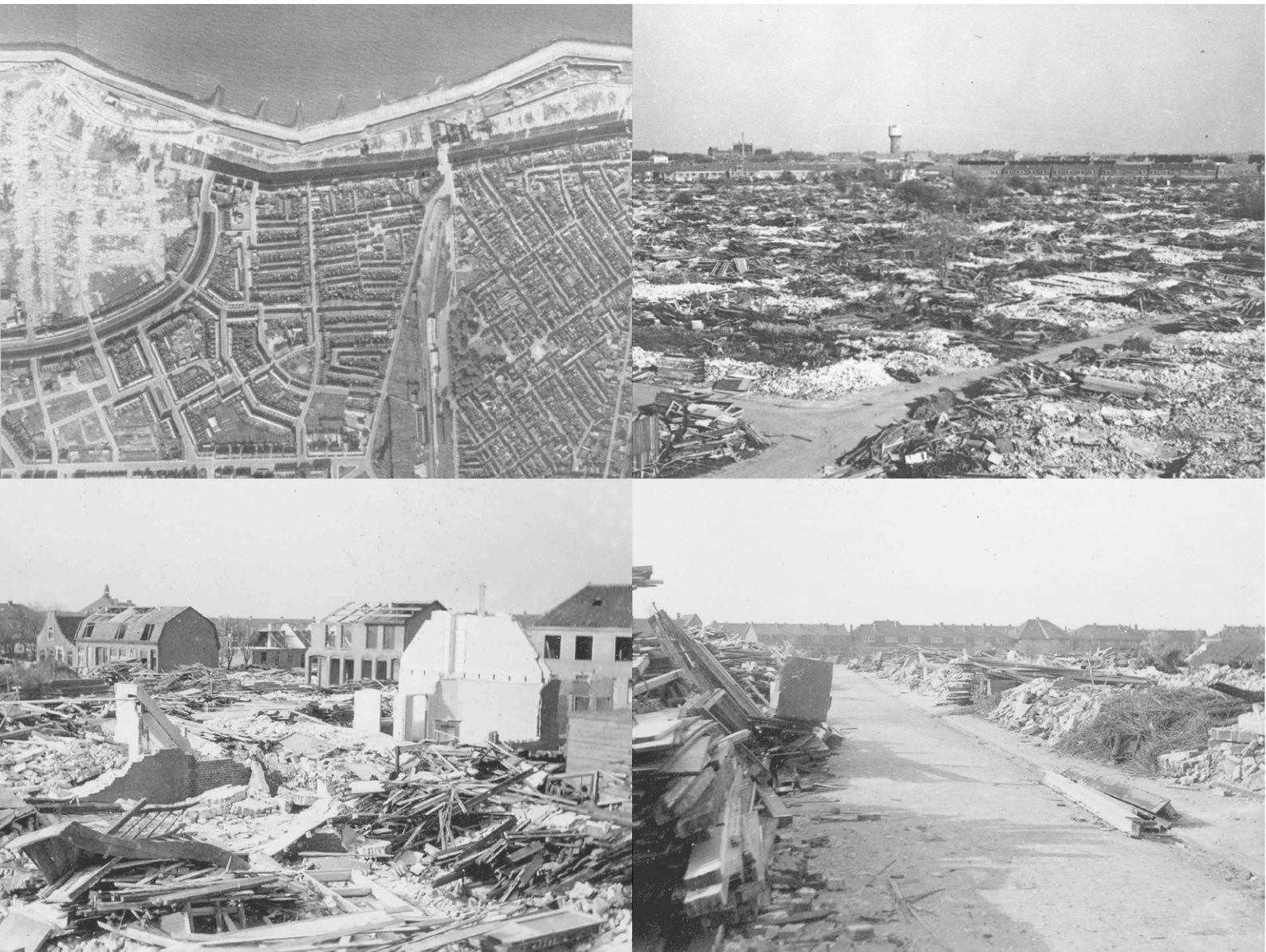
Figure 01-1 Photograph of the Den Helder demolition zone in 1942 Source: WUR Library Special Collections, and Den Helder Historical Society
