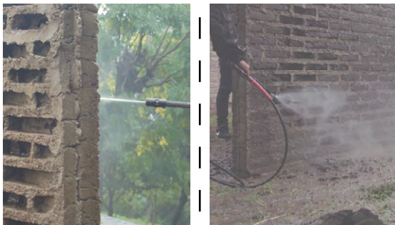
bricks were pushed out with pressure washers
