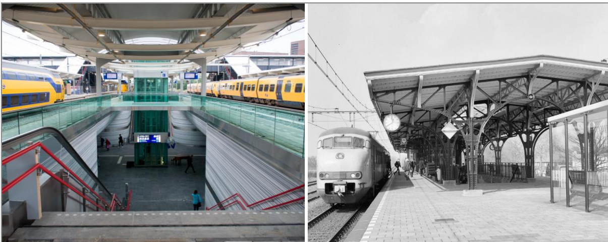
Figure 13: Left: Railway tunnel Zwolle (Wever, 2015). Right: Platform canopy at station Geldrop (Heins, 1997)
