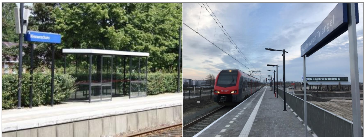
Figure 16: Left: Waiting shelter at station Nieuweschan. Right: Station Waddinxveen Triangel with no form of shade present. (ProRail, 2018c)
