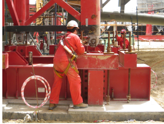
Figure 17: Base frame on foundation (Mammoet).
