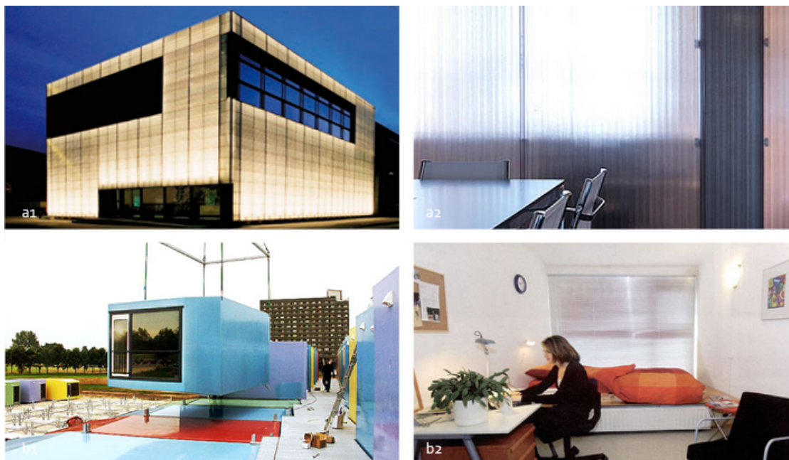
Figure 8: a1. A lightweight ( 14 \text{ kg/m}^2 ) GFRP façade and a2. Its interior (source: www.scobalit.ch/pdf/scobanews ), b1. A self-bearing GFRP sandwich composite modular house and b2. Its interior (source: mocoloco.com/archives )
