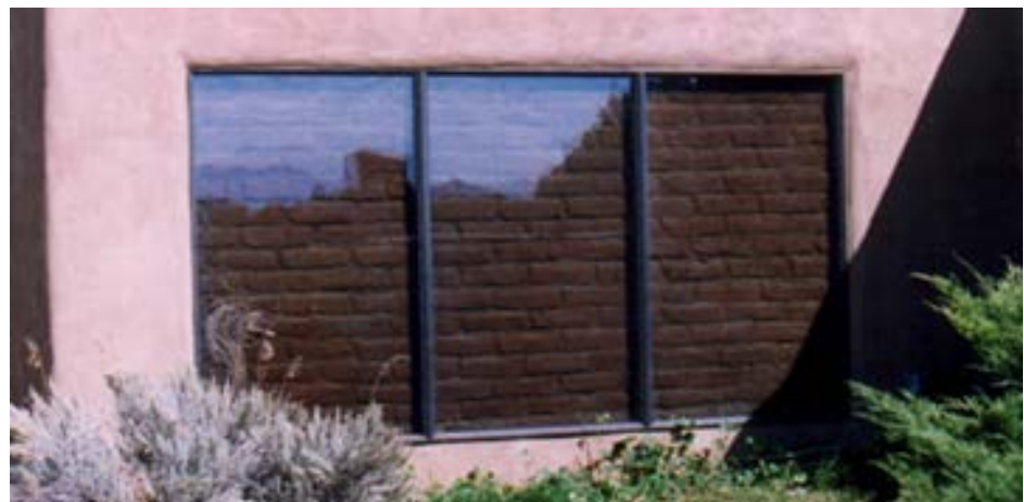
Figure 84: Exterior View of a Trombe Wall (source: http://www.lxrdesign.biz/DETAILS.htm )
