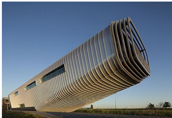
Figure 5: Lightweight Steel Frame and Cladding to assist a large cantilever (source: Wilo Nederland industrial building, Westzaan (Bentham Crouwel Architects))
