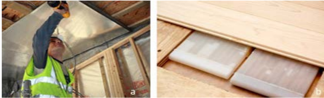
Figure 4: a. Installation of an ENERGAIN PCM panel at a wooden building's ceiling (source: www.offsite2007.com/progress-photos ) b. Installation of Deltacool PCM panels at a wooden building's floor (source: www.webtarry.com/ideas )
