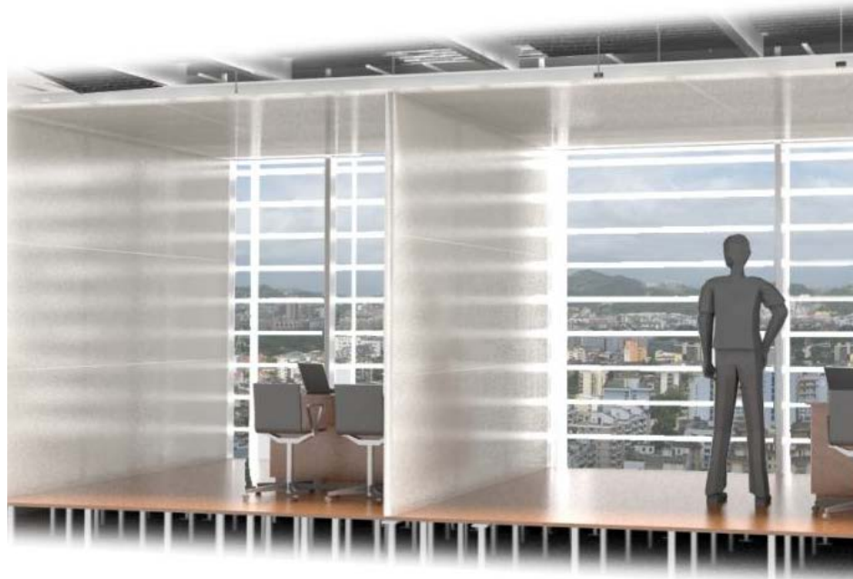
Figure 77: Epoxy panel A with CLIMASEL PCM at an office, at ceiling and walls, during day.
