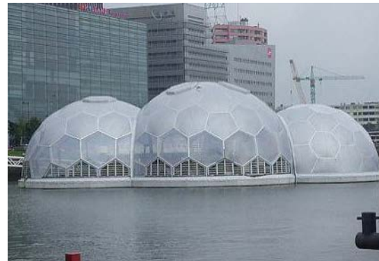
Figure 6: Lightweight Steel Frame and Cladding to assist floatation (source: Floating Pavilion, Rotterdam (Public Domain Architects and Deltasync))
