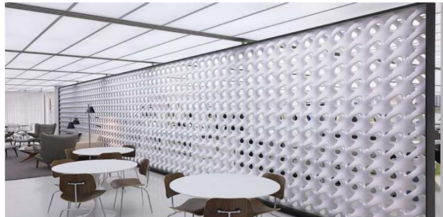
Figure 91: Casted gypsum-cement partition wall, designed by Erwin Hauer, at ElieTahari's Manhattan fashion studios, NY (source:www.erwinhauer.com)
