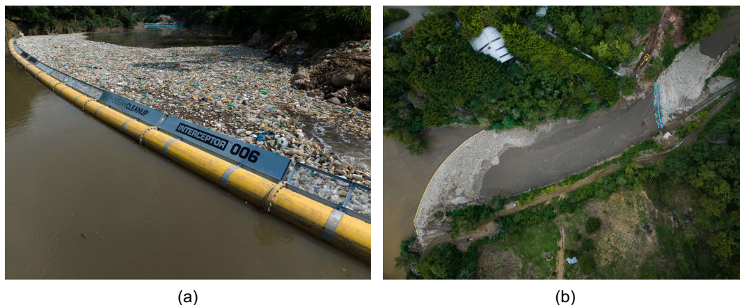
Fig. 1. Accumulation of plastic debris at waste-collection devices, creating the so-called carpet : (a) plastic debris captured by the floating boom, looking at upstream direction; and (b) aerial view of the carpet formations upstream of the waste-collection device. (Images courtesy of The Ocean Cleanup.)
