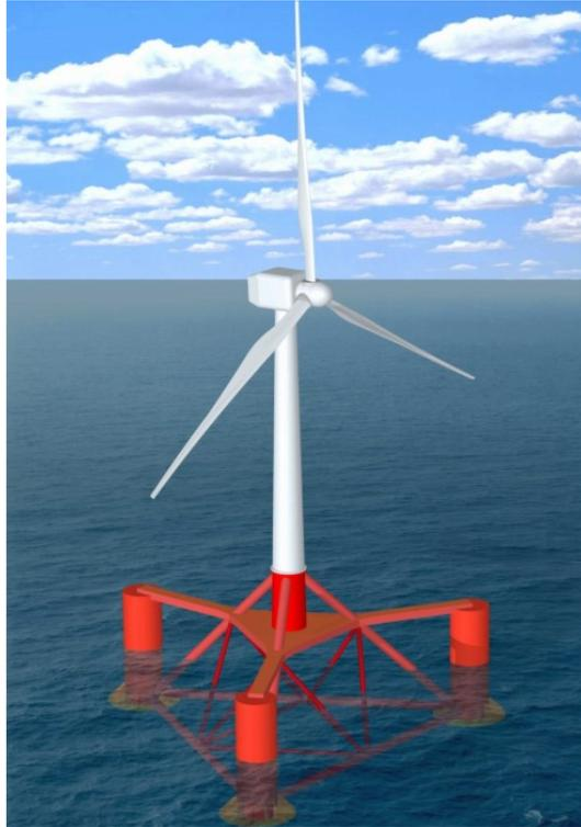
**Figure 2-5:** A semi submersible type floating wind turbine [6]. Based on the offshore experience of the petroleum industry, this design combines the mechanisms for stability.
