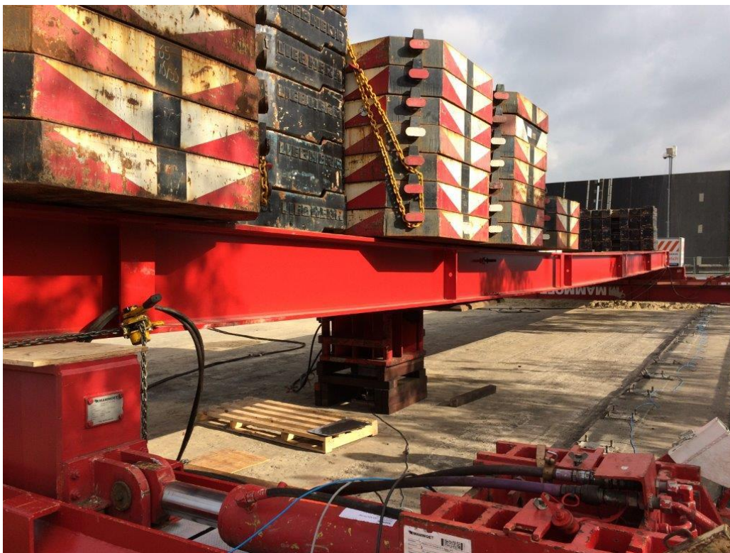
Figure 15. Use of counterweights, steel spreader beam, and a single hydraulic jack.
