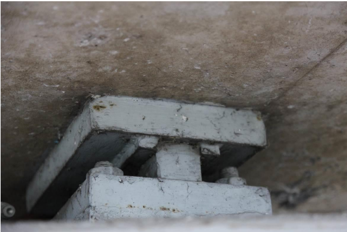
Figure 1. Example of frozen bearing.
