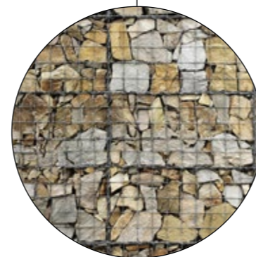
Fillable gabion walls
