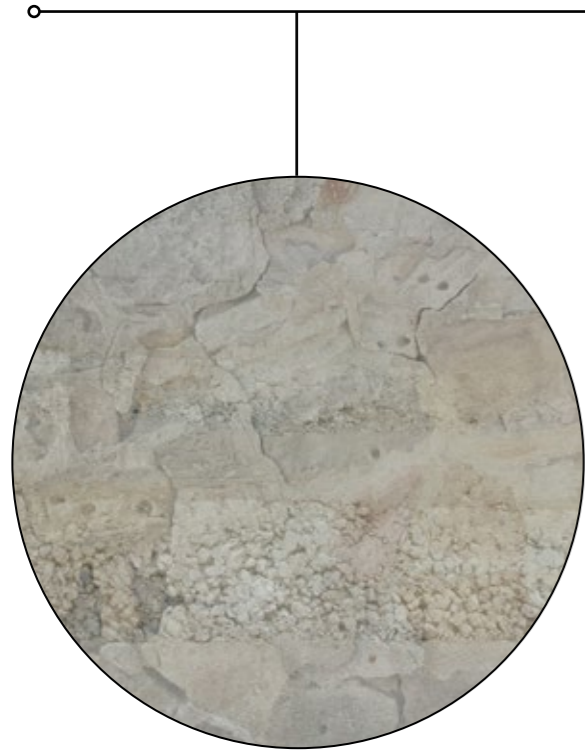
Rammed earth walls with larger aggregate - carving possibilities
