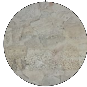
Rammed earth walls with larger aggregate - carving possibilities
