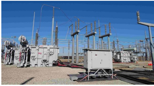
(a) Siemens 345/115 kV, 400 MVA Autotransformer[26]
