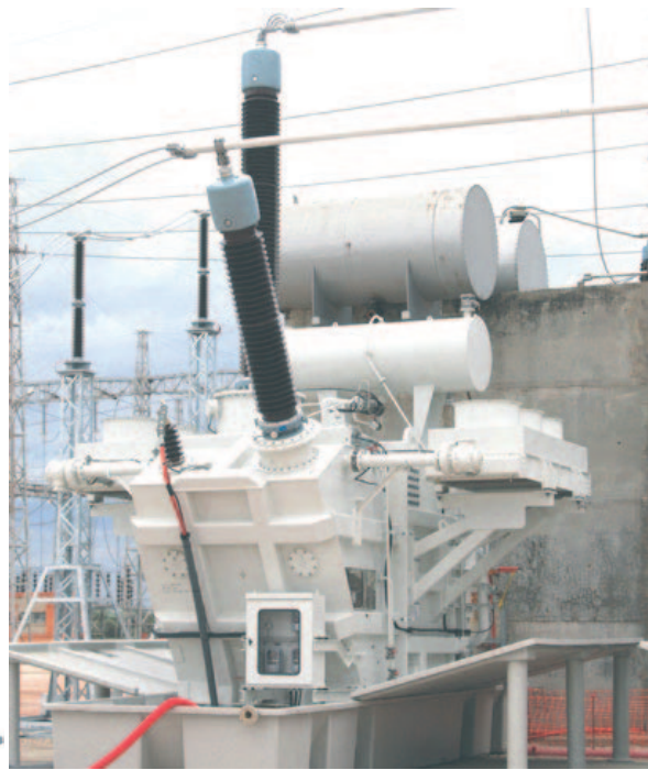
(b) ABB mobile transformers single-phase in operation [4]
