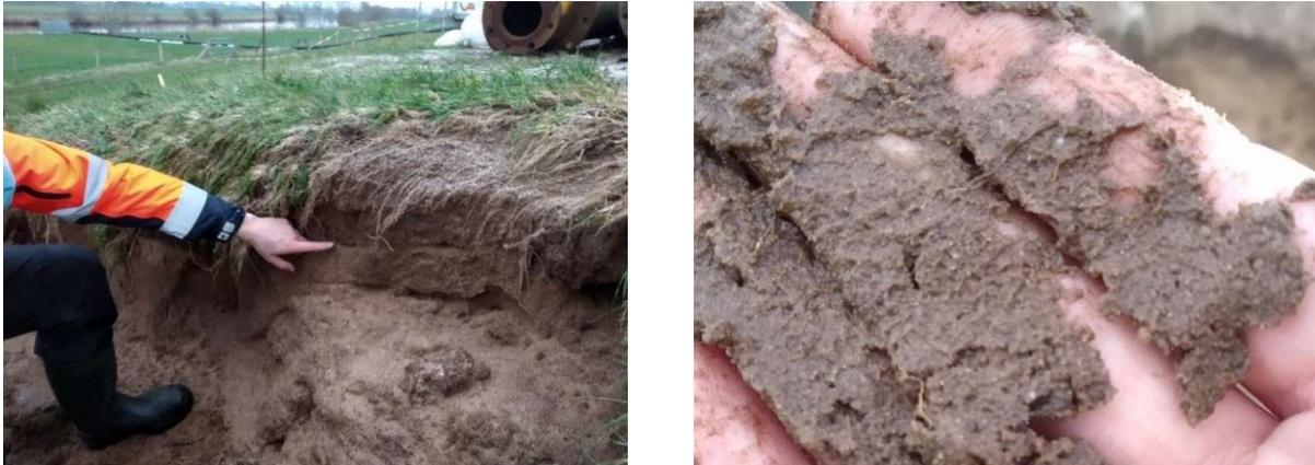
Figure 8 "Interne slemp" at the Vechtdijk, 2021. Left: Location of erosion resistant layer. Right: Material in this layer.
