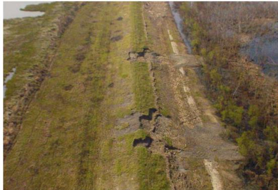
*Figure 1 Example of the vulnerability of levee landside slopes to external erosion, from the New Orleans East Basin (USACE, 2006).*
