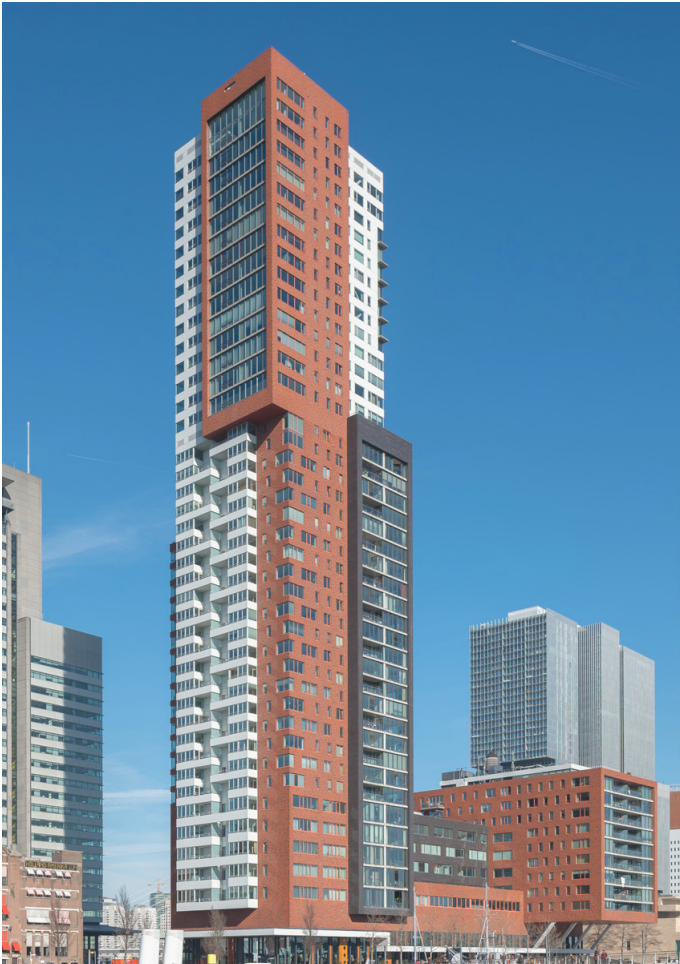
Figure 8.2 | Front view photo of the Montevideo. The light parts of the facade are the light grey cassettes, which are the focus of this case study | Source: (Mecanoo 2021)
