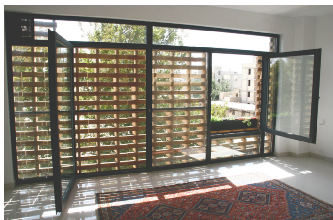
Figure 4.9 | Photograph of an example of a 'Mashrabiya' applied in a high-rise building | Source: (designboom, 2012)
