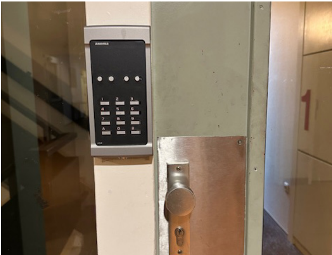
Image 34. Lock on an exit (own work)
