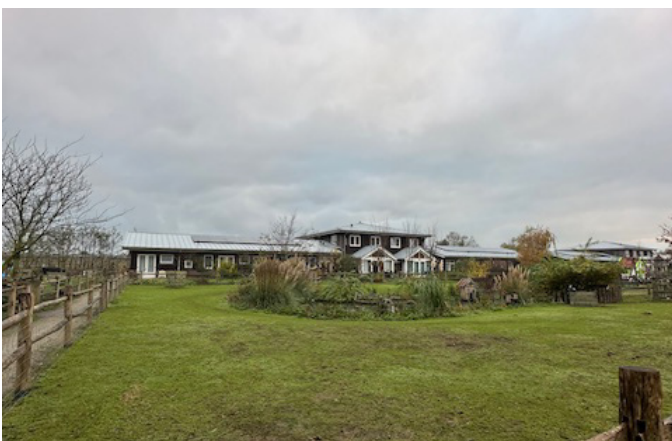
Image 89. Part of the inner courtyard (own work)
