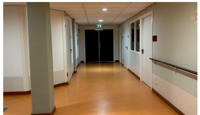
Image 16. Dead end + railings (own work)
