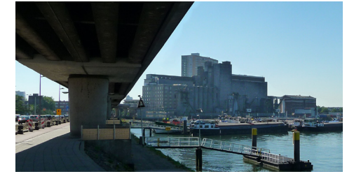
104. The Viaduct and the Maassilo. Source: by the author, 2012
