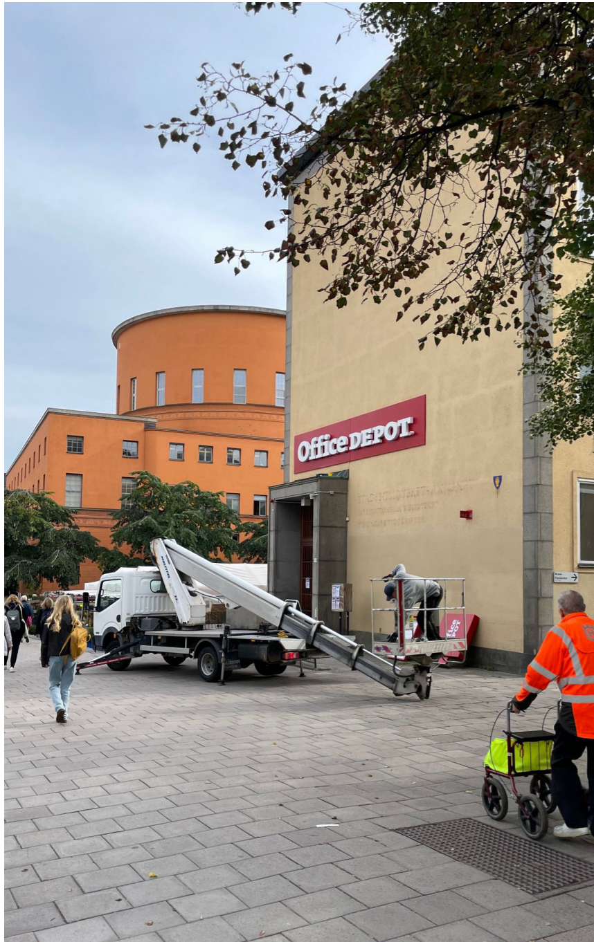
Annex 01 1952 - Humanities Library 2024 - Office Depot
