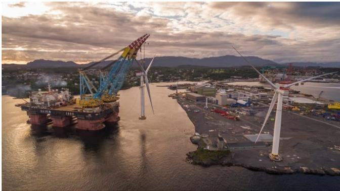
(c) Sheltered water strategy example of SAIPEM's S7000 lifting a WTG from the quayside to later install it on a floating support structure in the sheltered waters [95]. Multiple turbines are built up on the quayside awaiting their turn for the mating operation.
