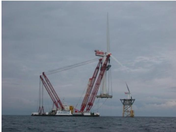
**Figure 2.7:** The lifting configuration used for the installation of the Beatrice Wind Farm Demonstrator Project [84].
