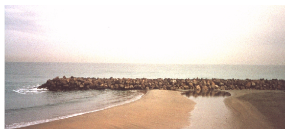
Fig. IV-3. Breakwater and induced tombolo
