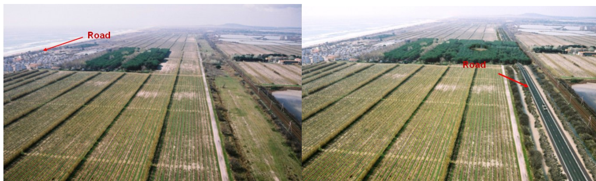
Fig. IV-17. Road realignment along the railways (site of Mas de Castellás )
