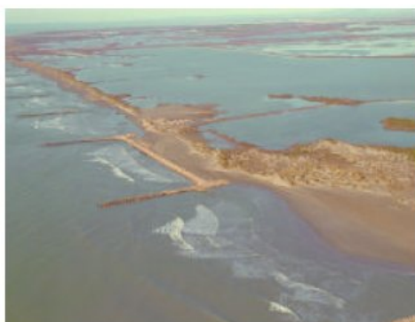
Fig. II-1. Flooding Petite Camargue (source EUROSION)
