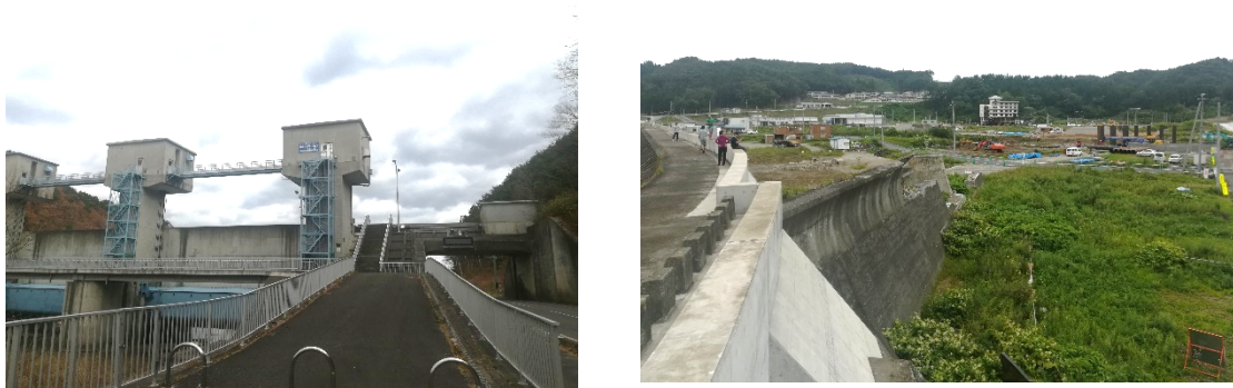
Figure 1. Left: The dyke and floodgates at Fudai successfully stopped the tsunami, despite suffering some overtopping (inundation marks of ~20m in front of the structure, indicated by
