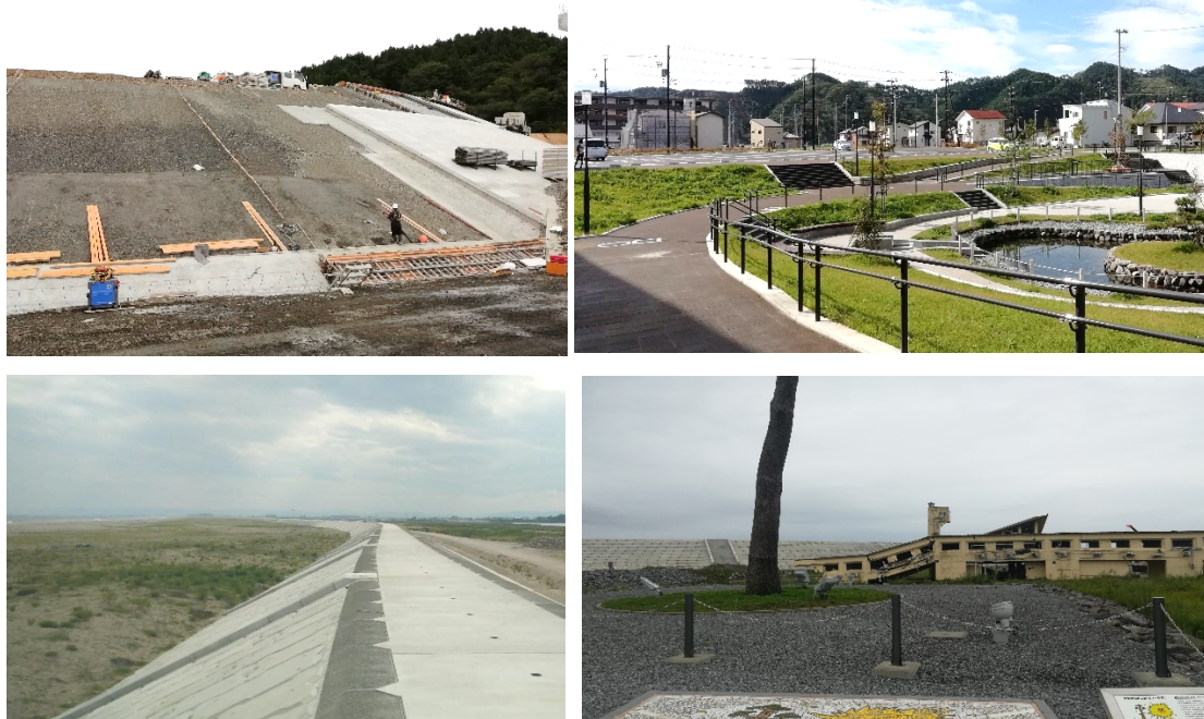
Figure 2. Top left. Construction of new dyke in Otsuchi town (Sept 2018). Top right. New park in Otsuchi, showing the original level of the town (pond on the right) and the new level (houses at the back). Bottom left. Reconstructed dike along the Sendai plains coastline (photo courtesy of Glasbergen, T). Bottom right. New coastal dyke at Rikuzentakata, in front of a preserved memorial building.
