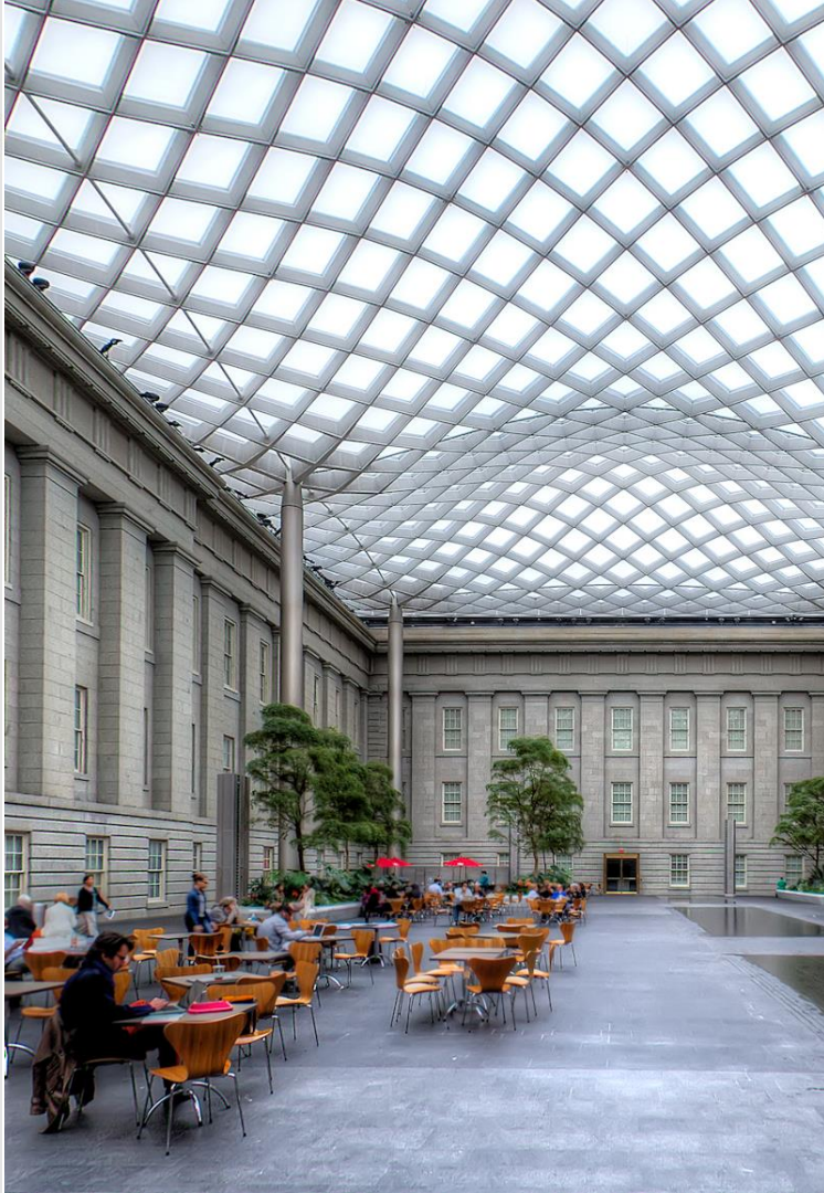
Figure 11. Translation surface covering two semi-circular plans connected with tangential edges.
