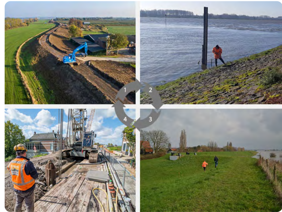
Figure 2: Example of the activities to ensure life-cycle performance: photo 1 and 4 reinforcement, 2 and 3 inspection. Photos by HWBP (2018, p.103) / Pascal Ogink, Wouter Jan Klerk, Mark van der Krogt and the Flood Protection Programme, respectively.
